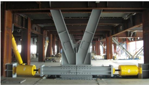
増幅機構付粘性減衰装置 Viscous Damping Device with Amplifying Mechanism
